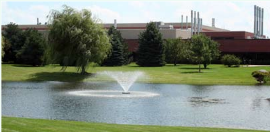
The property EMCO plans to purchase is located on the southeast corner of 95 th Street and 88 th Avenue. The site is the former home of Lawter International and Hexion Specialty Chemicals.
