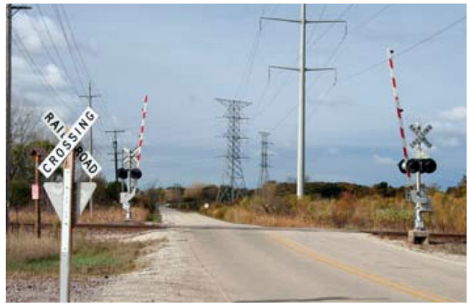
Image of the Union Pacific tracks as they cross Bain Station Road. The February 8 derailment occurred just north of the crossing.
